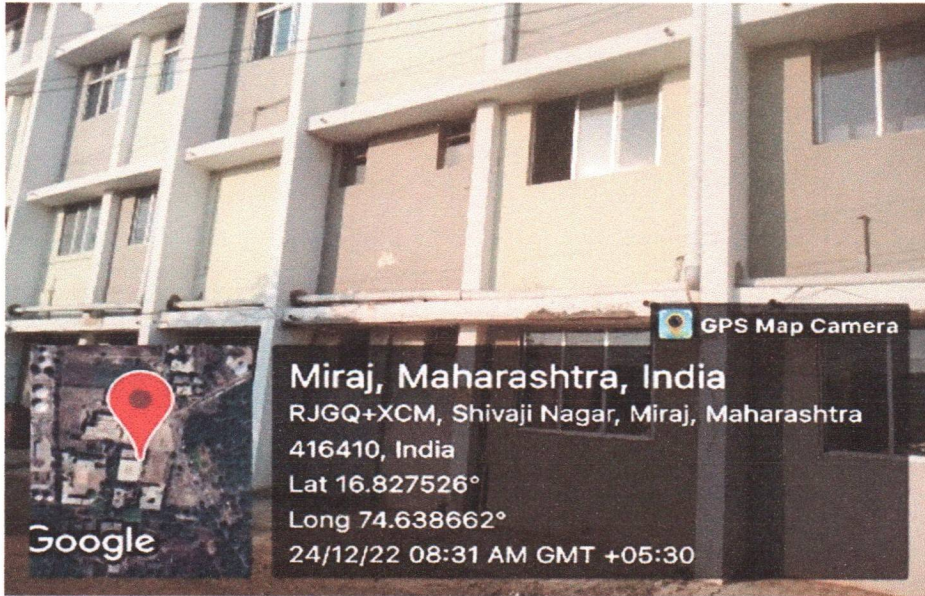
Rain water Harvesting system
